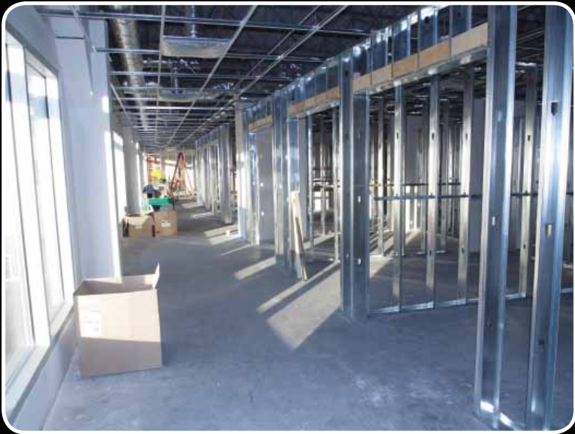
CONSTRUCTION UNDERWAY ON OUR NEW HEAD OFFICE ON OCTOBER 31, 2011
