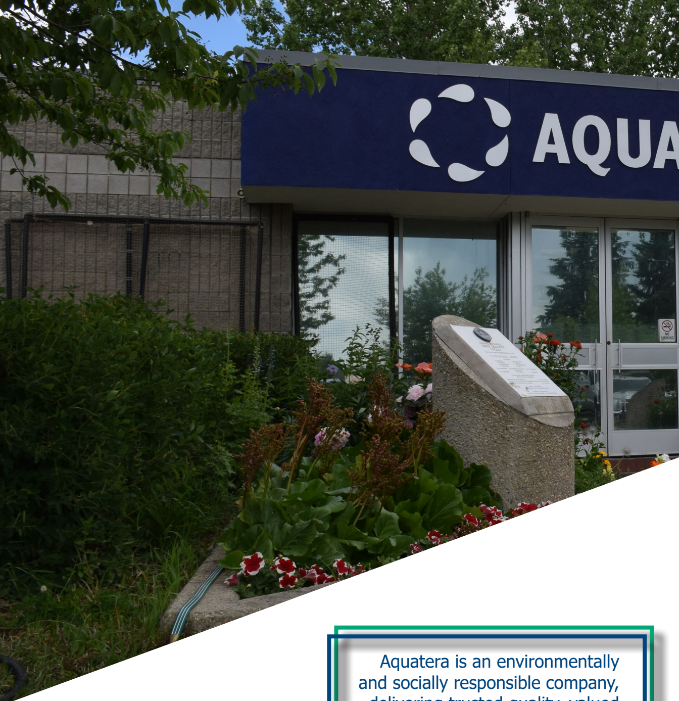
Photo of our Water and Wastewater Treatment Plant Administrative Building.
